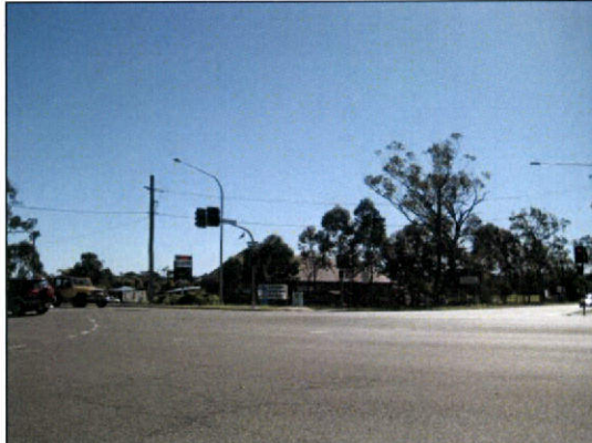
Photograph 3: View of "The Dam Hotel" diagonally opposite site to north-west.
