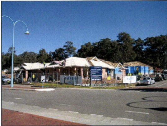
Photograph 7: View of group homes under construction by ADHC.
