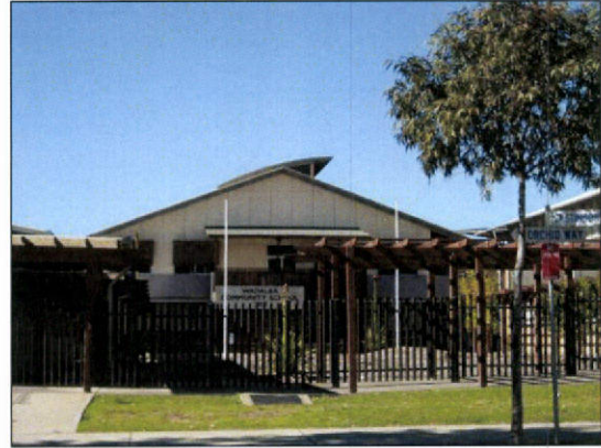
Photograph 8: View of entrance to Wadalba Community School at intersection of Orchid Way with Edward Stinson Avenue.
